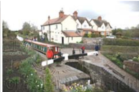
Canal Locks at Astwood Lane
