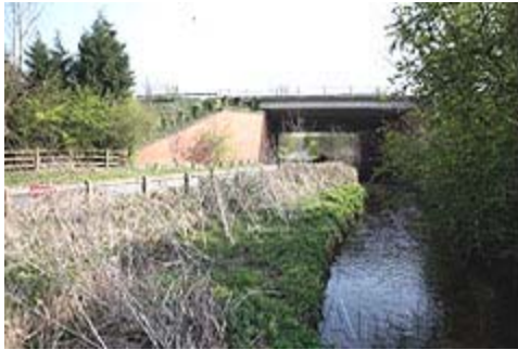
Crown Lane, bridge under the M5 Motorway
